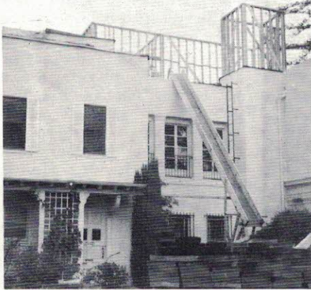
Library Penthouse being transferred into new offices.
